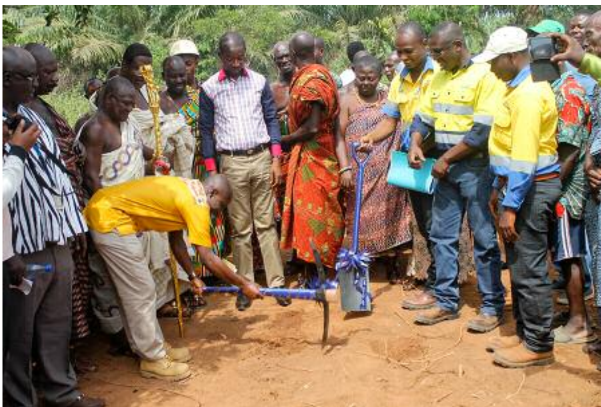
(Groundbreaking for the construction of six unit classroom block at Old Abirem)
