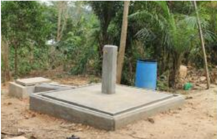
Hweakwae standpipe
