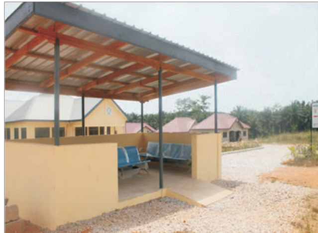
Waiting shed at Afosu Clinic
