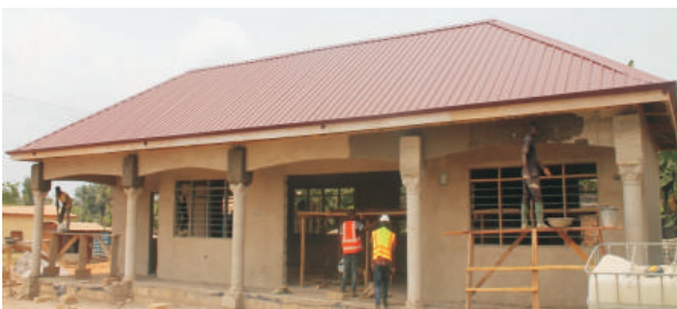
Construction of Conference Hall and out house at Mamanso durbar ground
