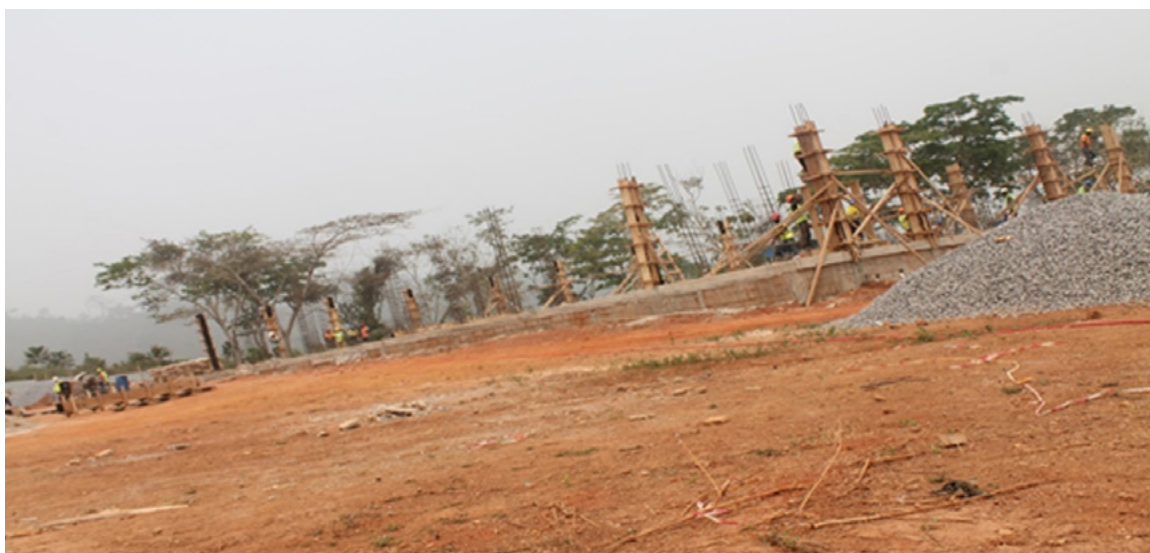
Picture 11: AVTI Construction
