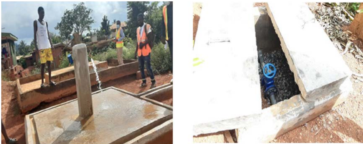
Picture 20 - One of the standing taps and a chamber in Adausena community
