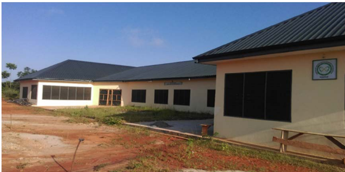
Picture 18 - Status of the new OPD as at 31st December 2021
