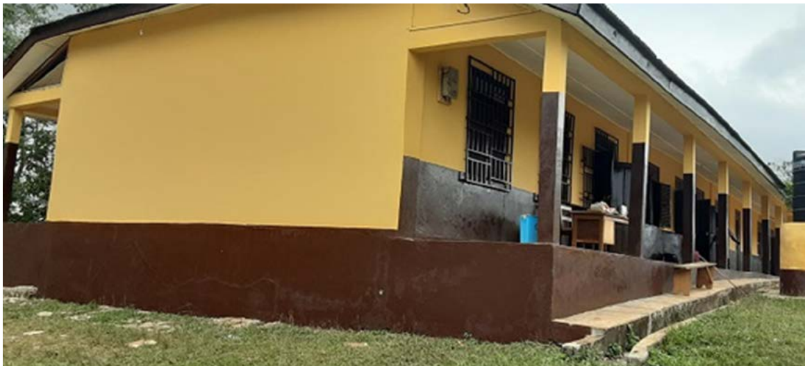
Picture 34 - Renovation of 1No. 4-Unit Classroom and Store at Adausena JHS
