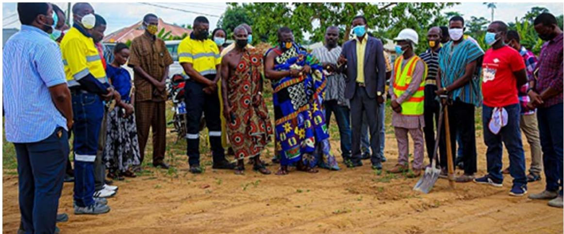
Picture 32 - Sod cutting for the New Abirem projects
