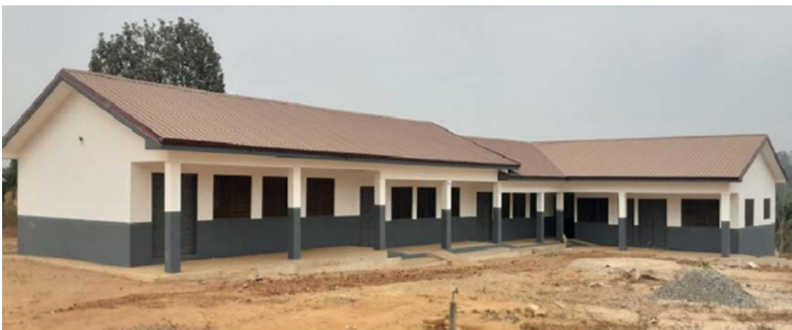
Picture 9 - 1No. 3-Unit classroom, office store and multipurpose room at New Abirem
