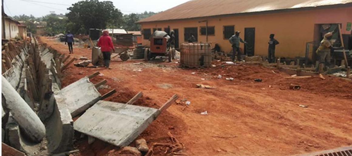
Picture 29 - Ongoing road construction in Afosu
