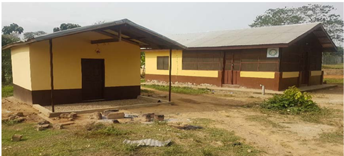
Picture 39 - Renovation of Hweakwae R.C. Primary School
