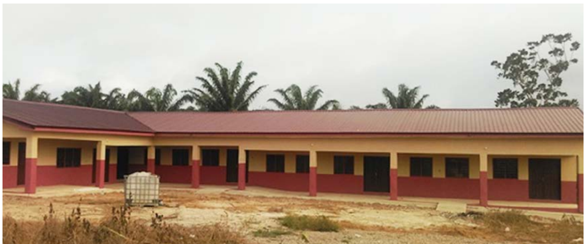
Picture 33 - 1No. 3 Unit Classroom, office, store and multipurpose hall at Mamanso.
